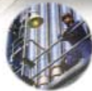
LV, MV and HV onshore cables for instrumentation, compensation, control and power
